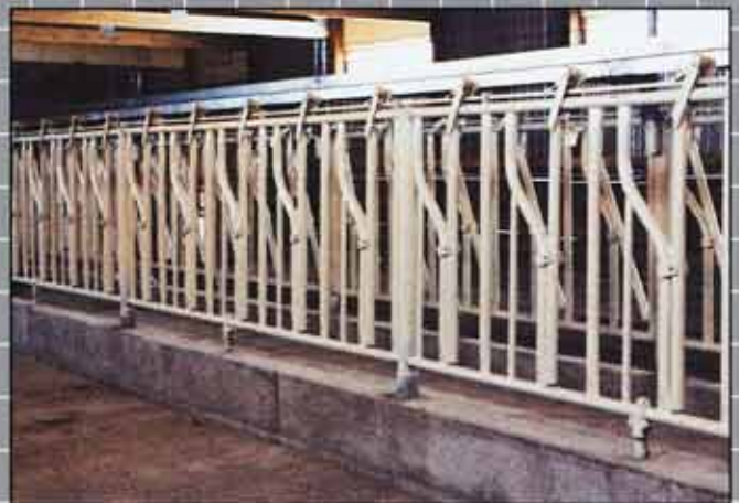
Weld between Steel Posts
